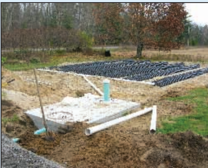
Leaching bed with gravelless trench technology.
