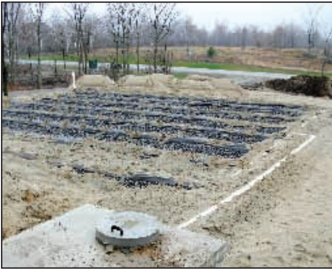
Leaching bed with perforated PVC drain pipes.
